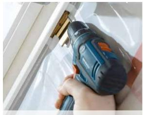
**3.** Install mounting clips to skylight drywall groove.
